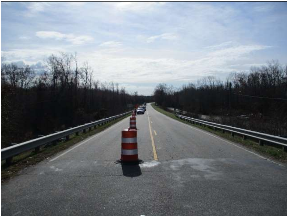
LOOKING SOUTH FROM BRIDGE
