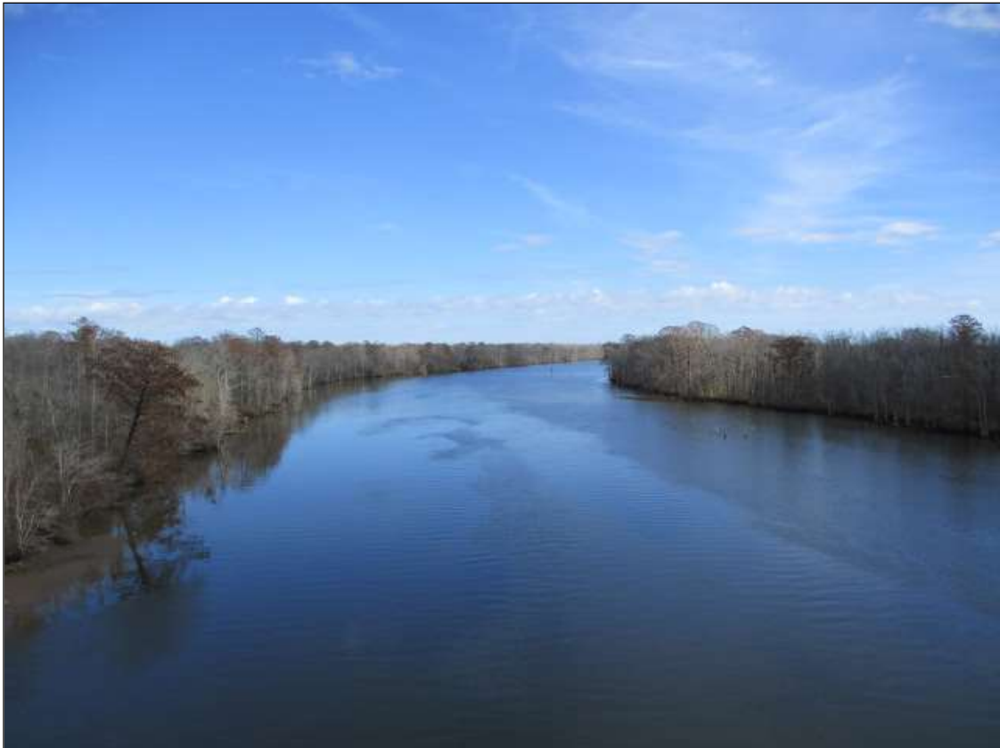
LOOKING EAST DOWNSTREAM AT SPAN 18 OVER THE ROANOKE RIVER
