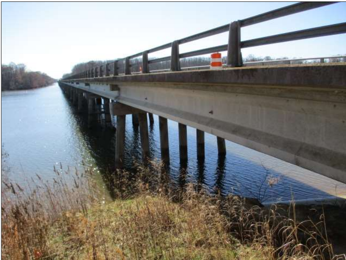
EAST ELEVATION FROM NORTH END
