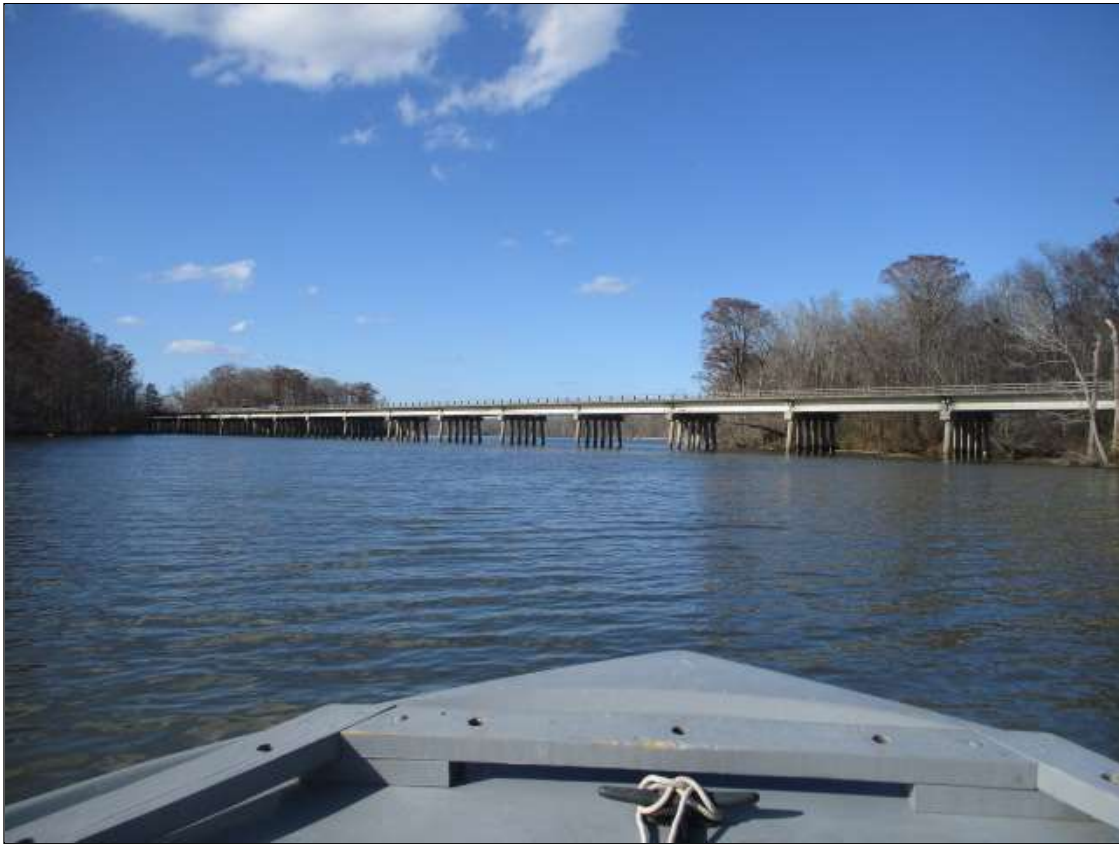
LOOKING EAST DOWNSTREAM OVER THE MIDDLE RIVER
