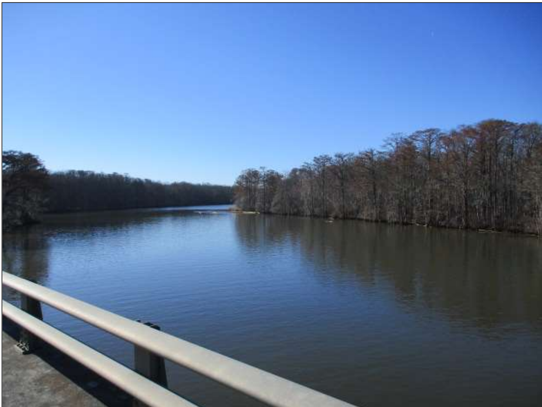
LOOKING WEST UPSTREAM AT SPAN 61 OVER THE MIDDLE RIVER
