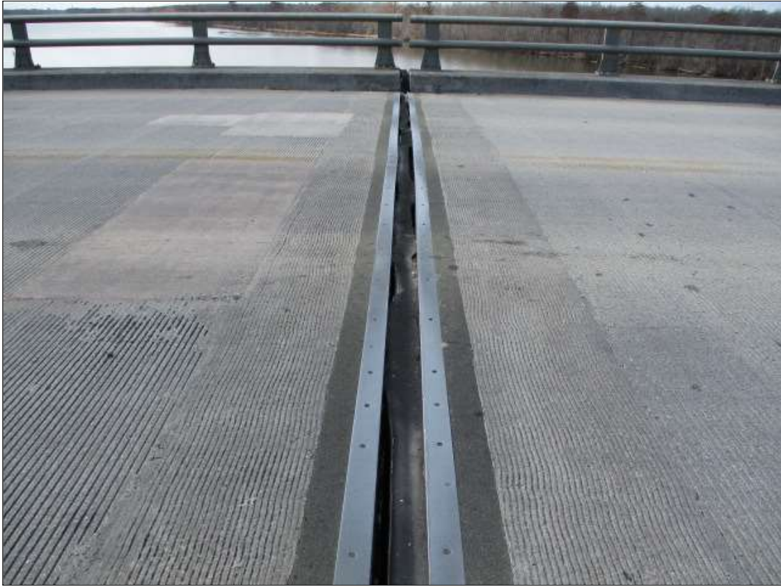
JOINT OVER BENT 16
