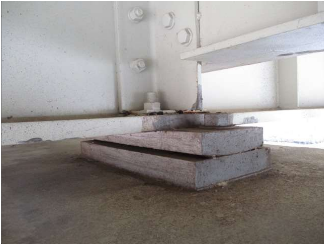
SPAN 17-19 INTERMEDIATE BEARING
