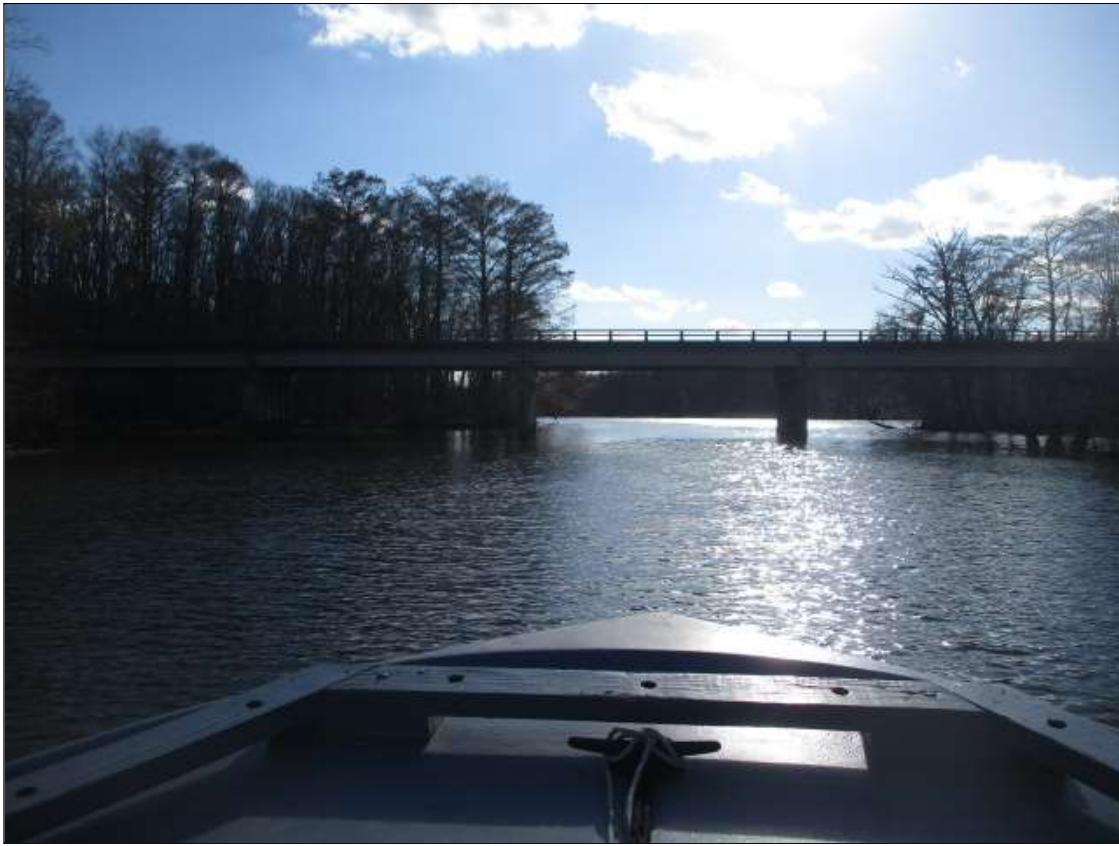
LOOKING WEST UPSTREAM OVER THE MIDDLE RIVER
