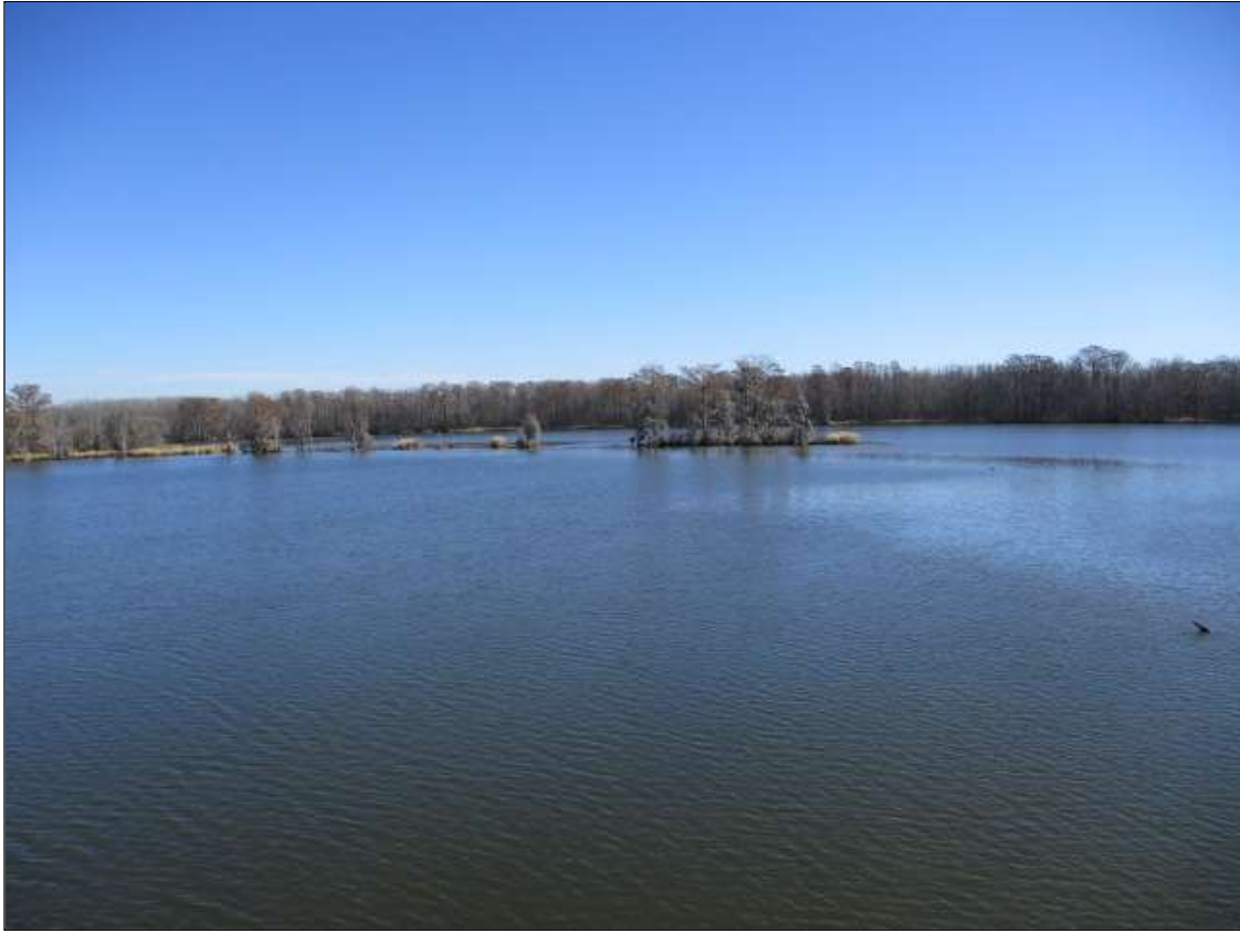
LOOKING EAST DOWNSTREAM AT SPAN 85 OVER THE CASHIE RIVER
