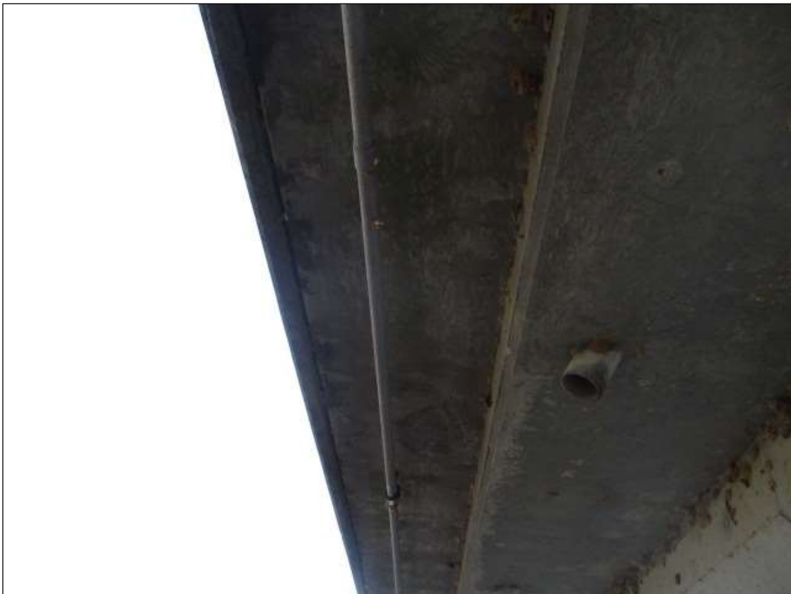
UTILITY IN LEFT OVERHANG
