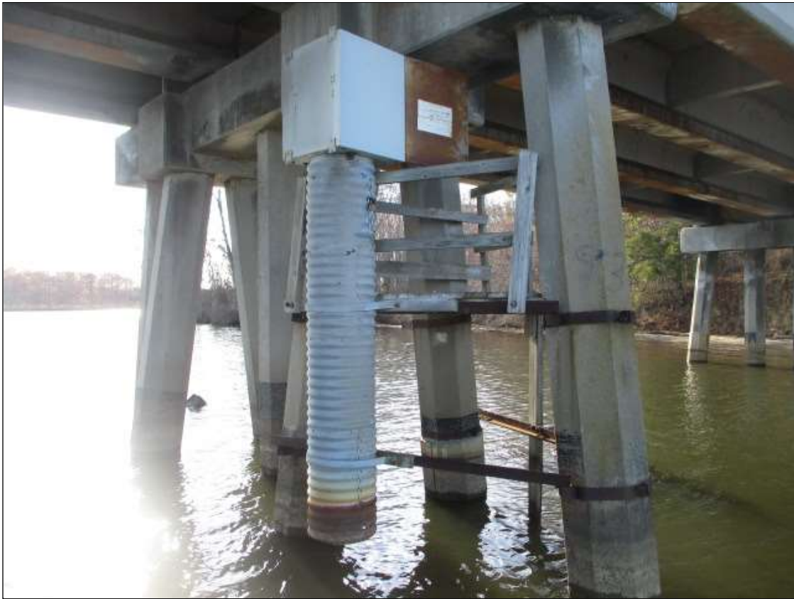
GAUGING STATION ON BENT 93 BETWEEN PILES 5/6 AND 7
