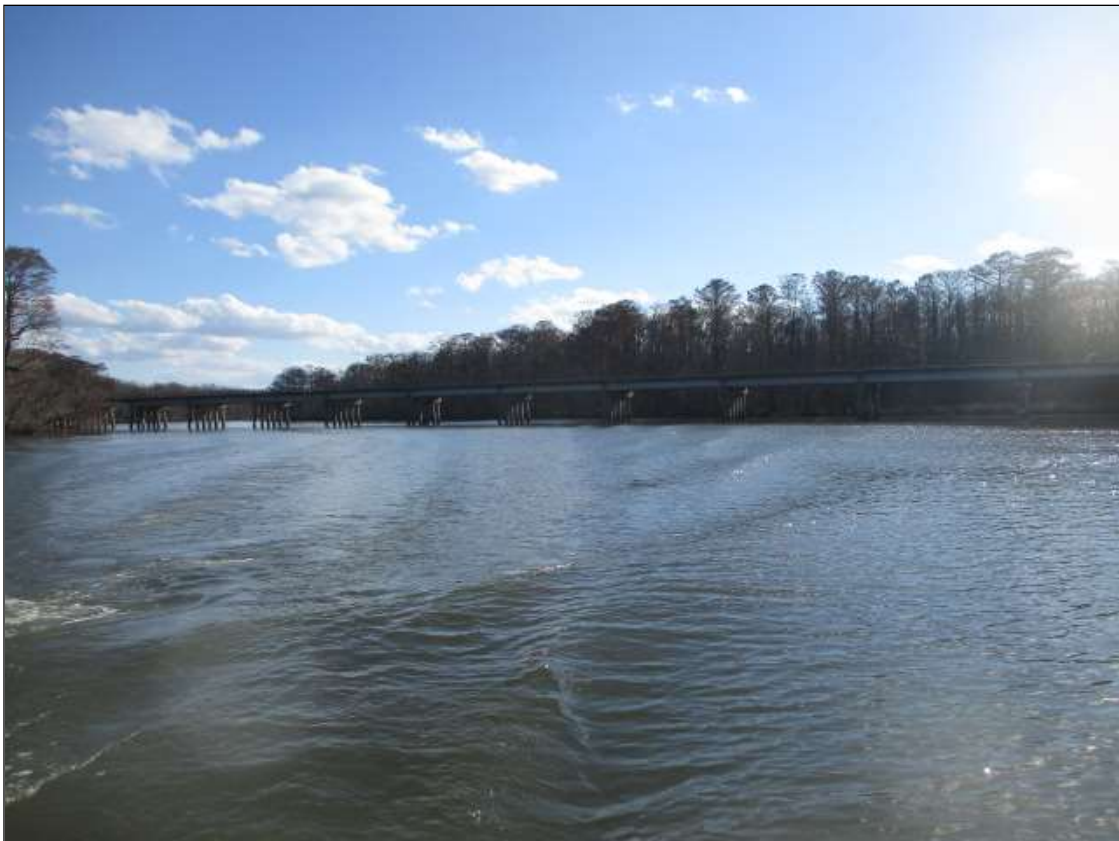
LOOKING WEST UPSTREAM OVER THE MIDDLE RIVER
