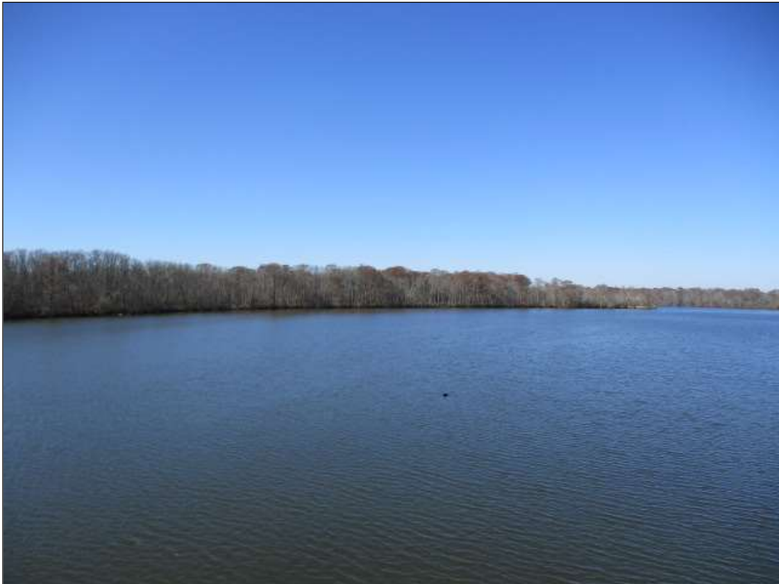
LOOKING WEST UPSTREAM AT SPAN 85 OVER THE CASHIE RIVER
