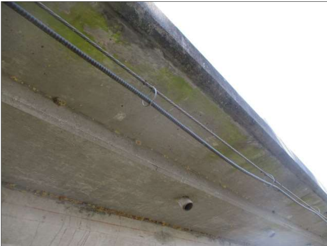
UTILITY IN RIGHT OVERHANG
