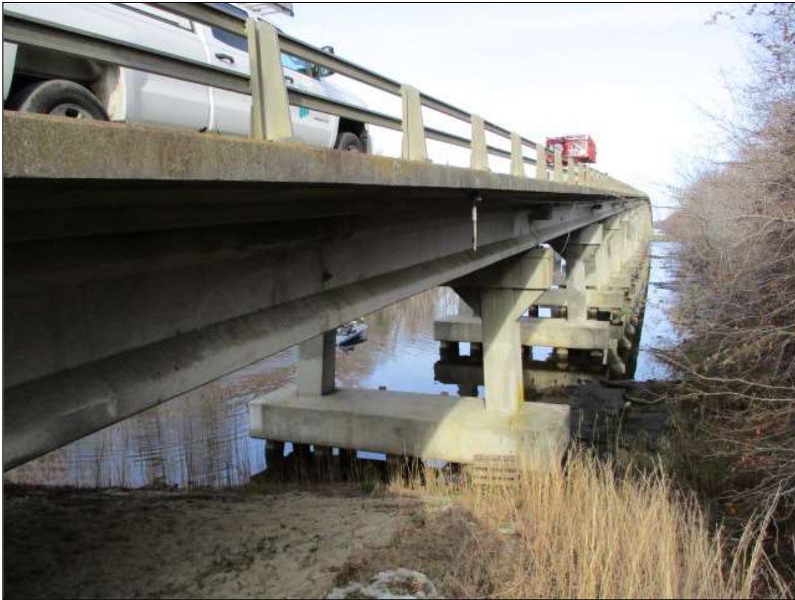
EAST ELEVATION FROM SOUTH END
