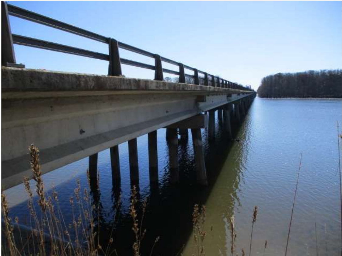
WEST ELEVATION FROM NORTH END
