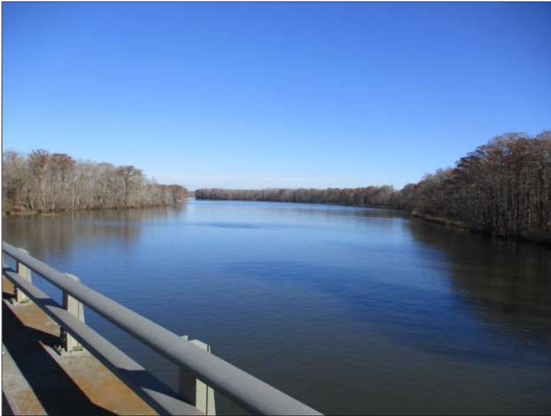
LOOKING EAST DOWNSTREAM AT SPAN 61 OVER THE MIDDLE RIVER
