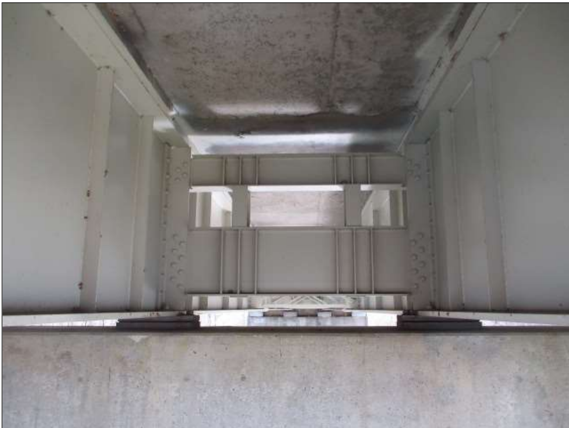
SPAN 17-19 END DIAPHRAGM
