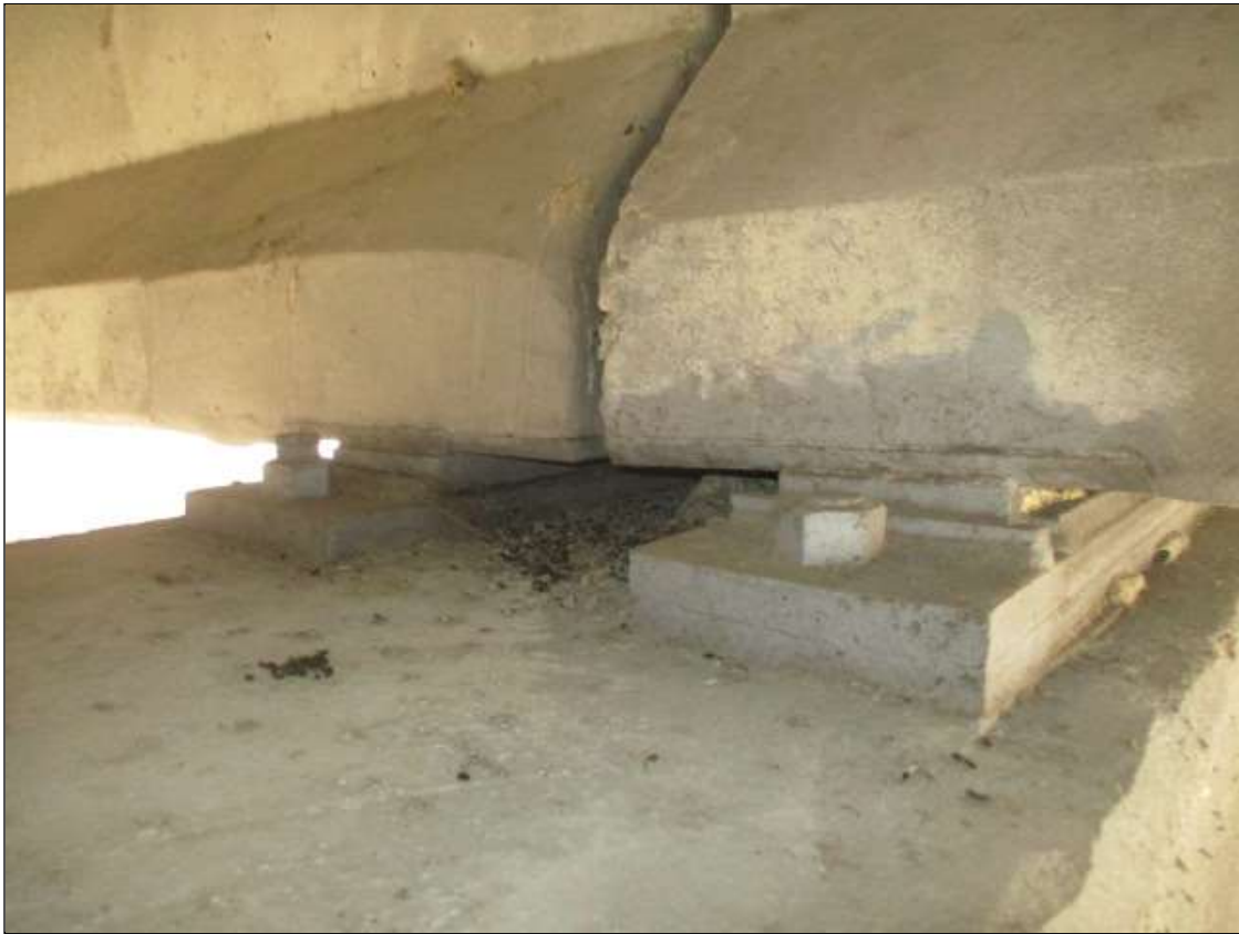
INTERIOR BENT BEARING
