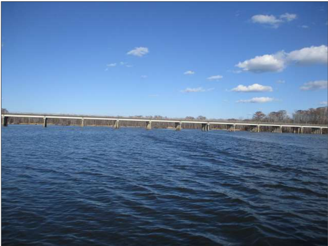
LOOKING EAST DOWNSTREAM OVER THE CASHIE RIVER
