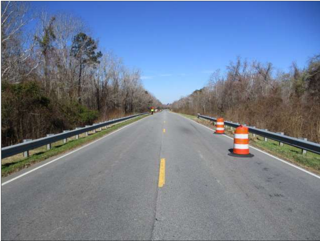
LOOKING NORTH FROM BRIDGE
