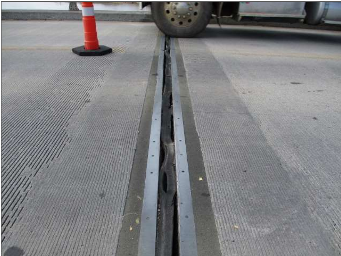
JOINT OVER BENT 19
